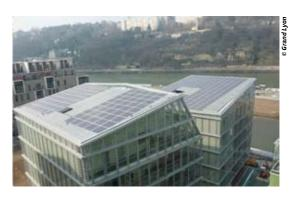
As it was difficult to ask each company in charge of the design and installation of a photovoltaic system to use the same monitoring system, a "district scale monitoring system" has been tailor-made to ensure that all PV systems operate properly on the long term.
